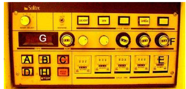
Main Control Panel
